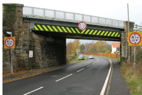
Warning chevrons and mandatory roundel signs showing the limit on vehicle height at a flat soffit bridge
