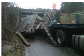
Bridge dislodged from abutments onto the vehicle which struck it
