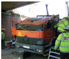
Crushed cab of a skip lorry following a bridge strike
